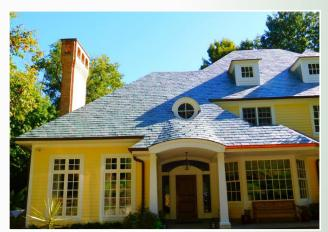
Slate Tile Roofing is common is older homes and higher-end construction. They offer a wide variety of colors, sizes, and installation patterns to add distinction and character to your home. Slate roofing is a durable, natural roofing product that has a long life-span if properly maintained.
